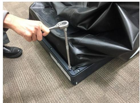
5. Pull the bars completely off the frame and set aside with the fasteners.
